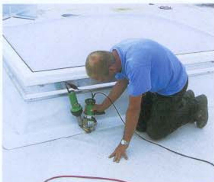
Welding of a membrane on a dome light.
