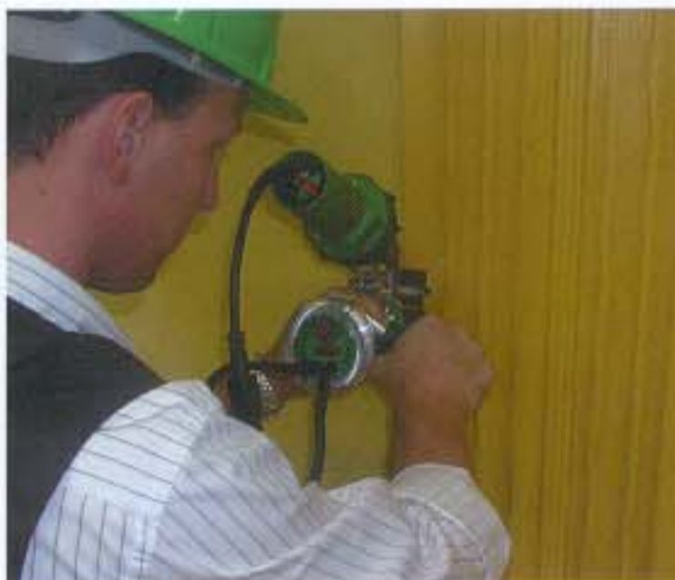
TriacDrive being used to weld a water bar in a tunnel.
