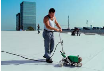
VARIMAT V used for overlap welding of plastic roofing membranes.
